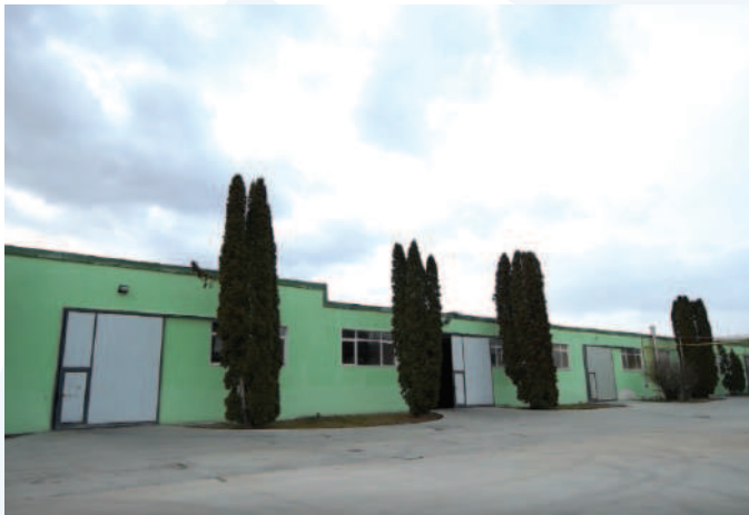
VISTA STABILIMENTO • PLANT VIEW
